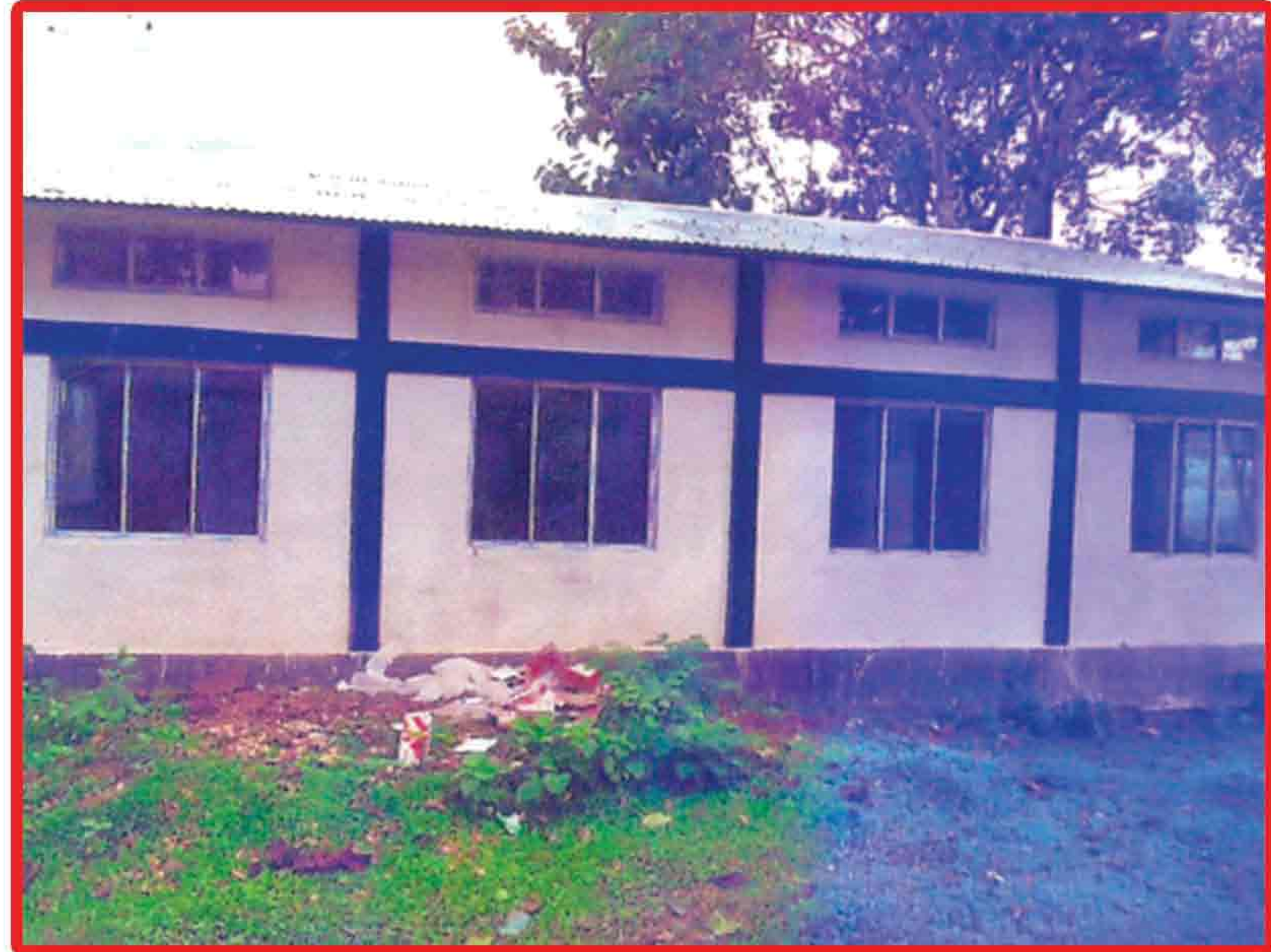
Const. of A.P. Building Extension At Patherkandi A.P.
