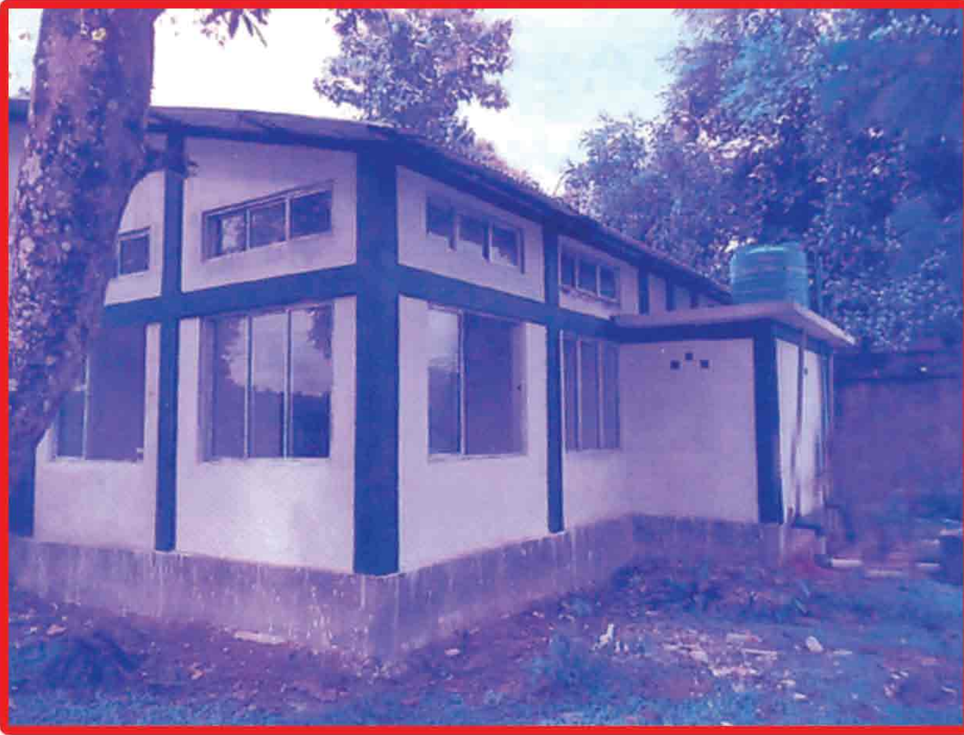
Const. of A.P. Building Extension At Patherkandi A.P.
