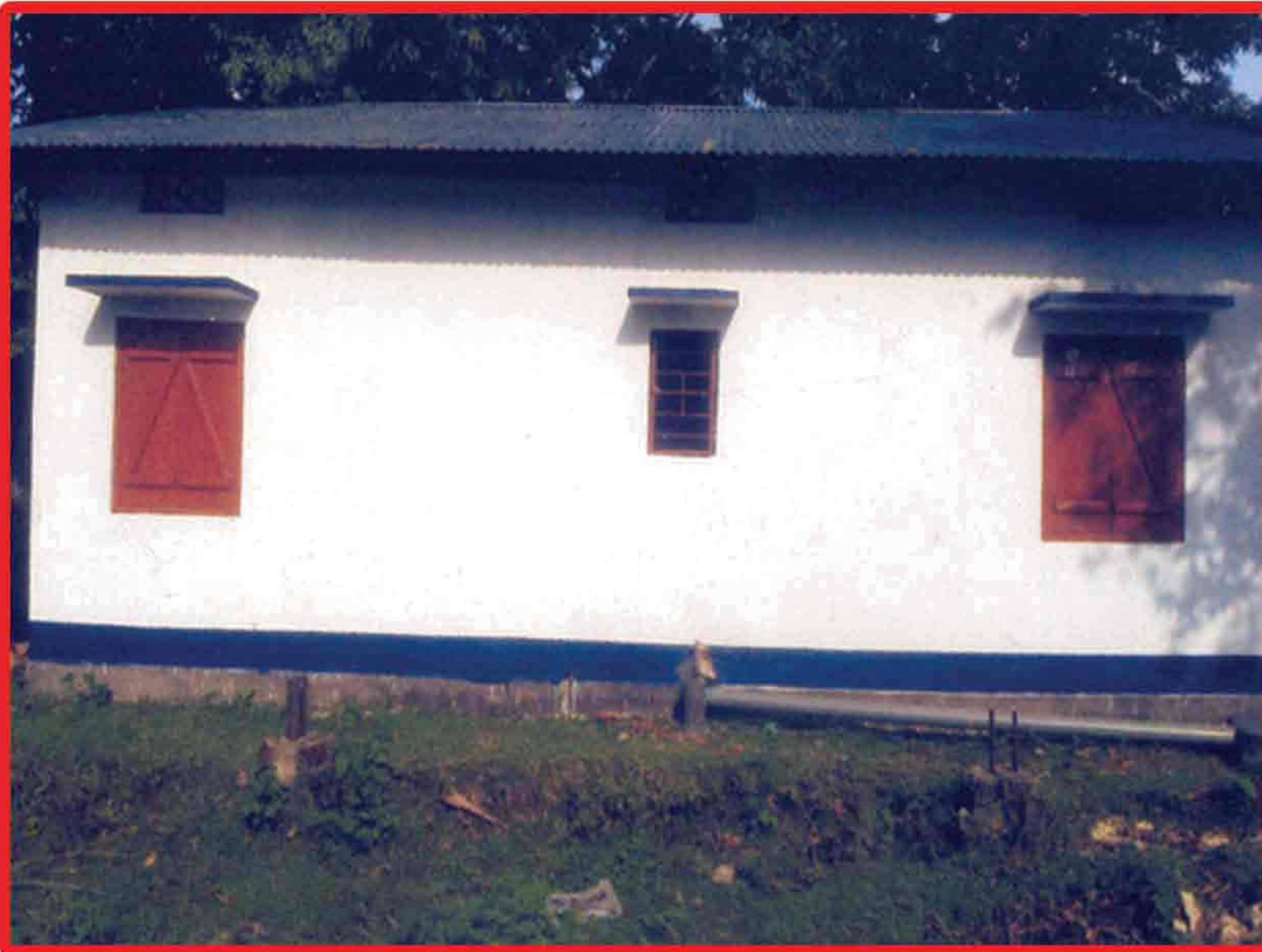
Construction of BDO/E.O Quarter at Badarpur A.P.
