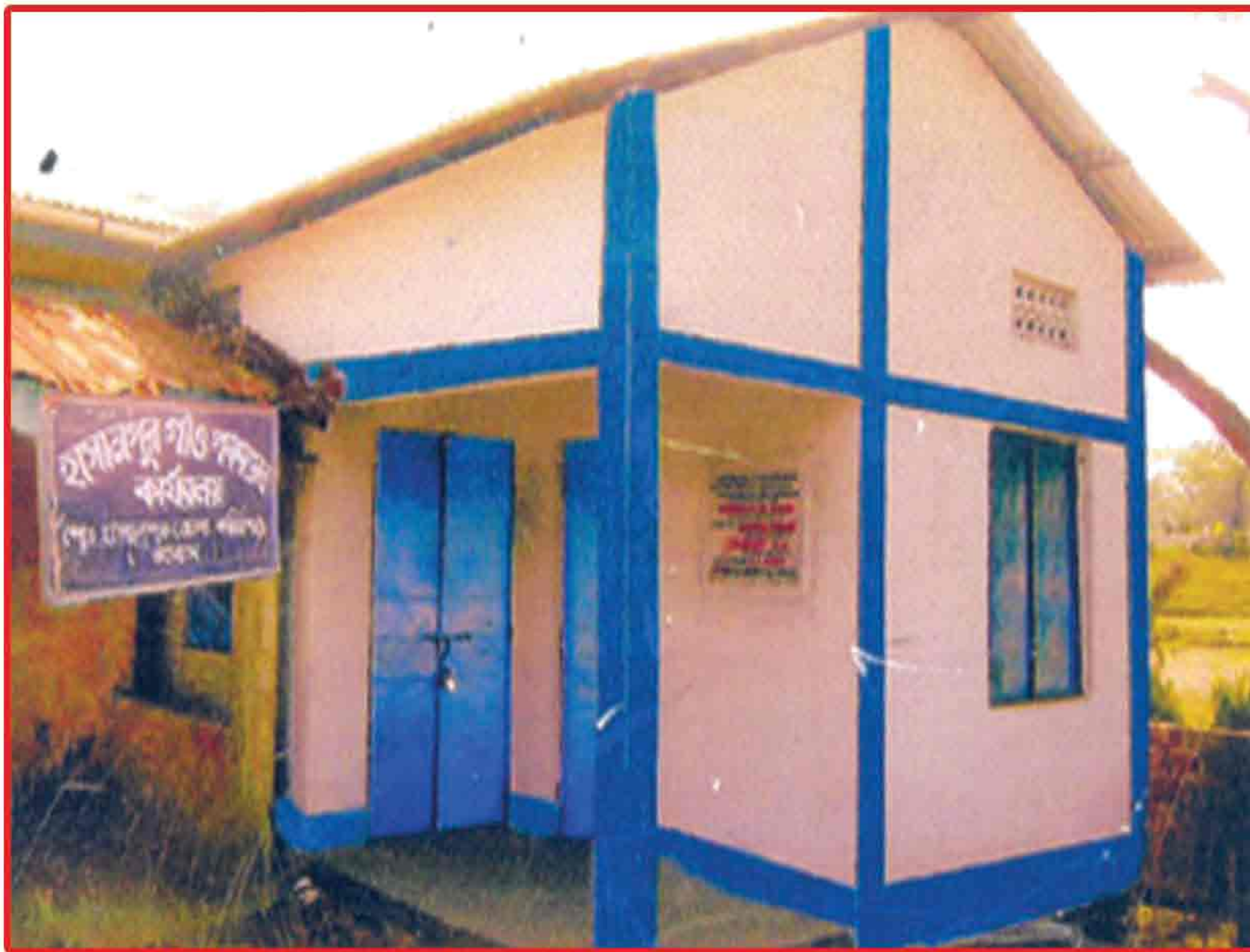
Construction of G.P. Secy Quater at Hasanpur G.P.
