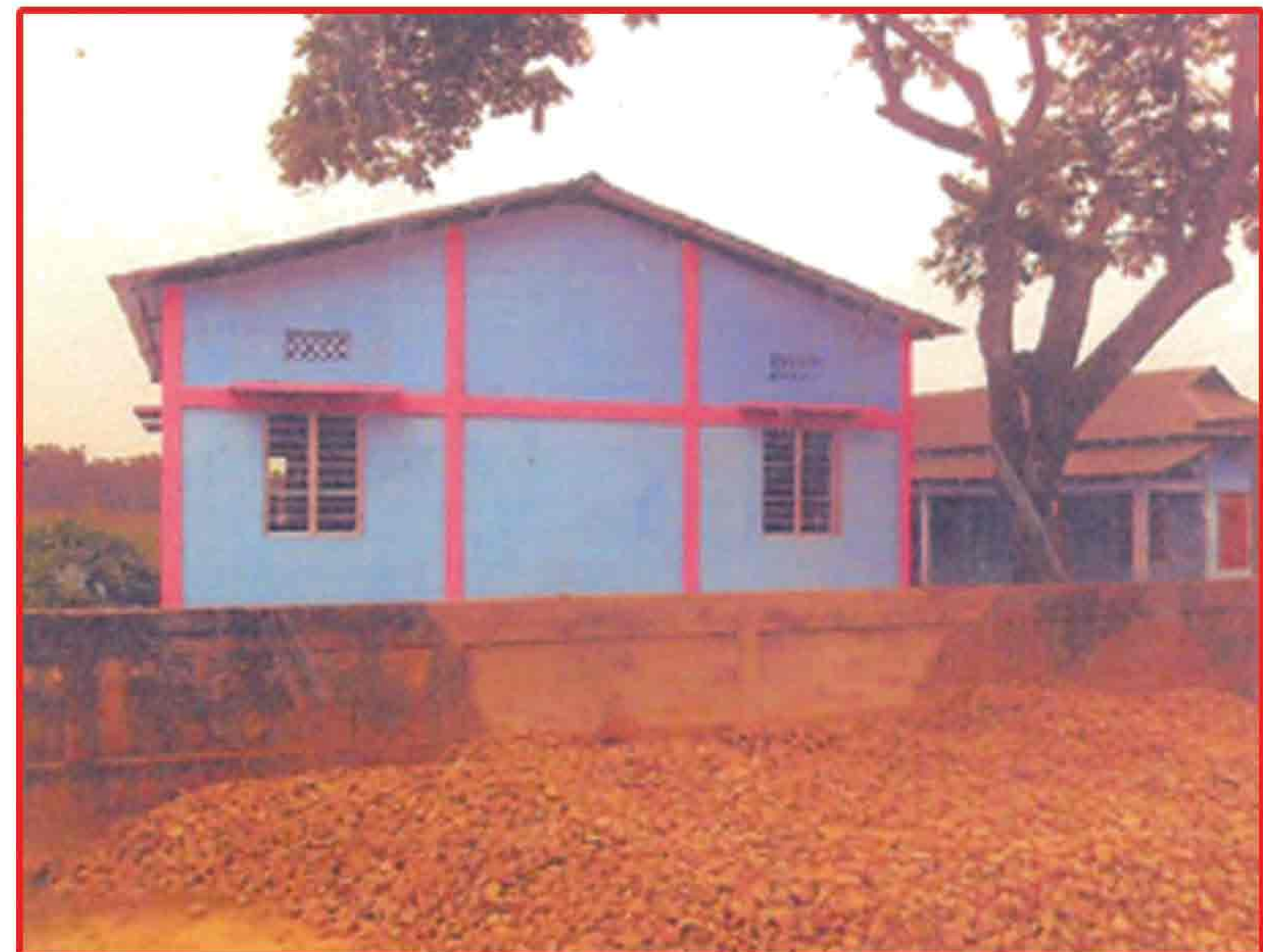
Construction of G.P. Office Building (Extension) at Pirarchak G.P.
