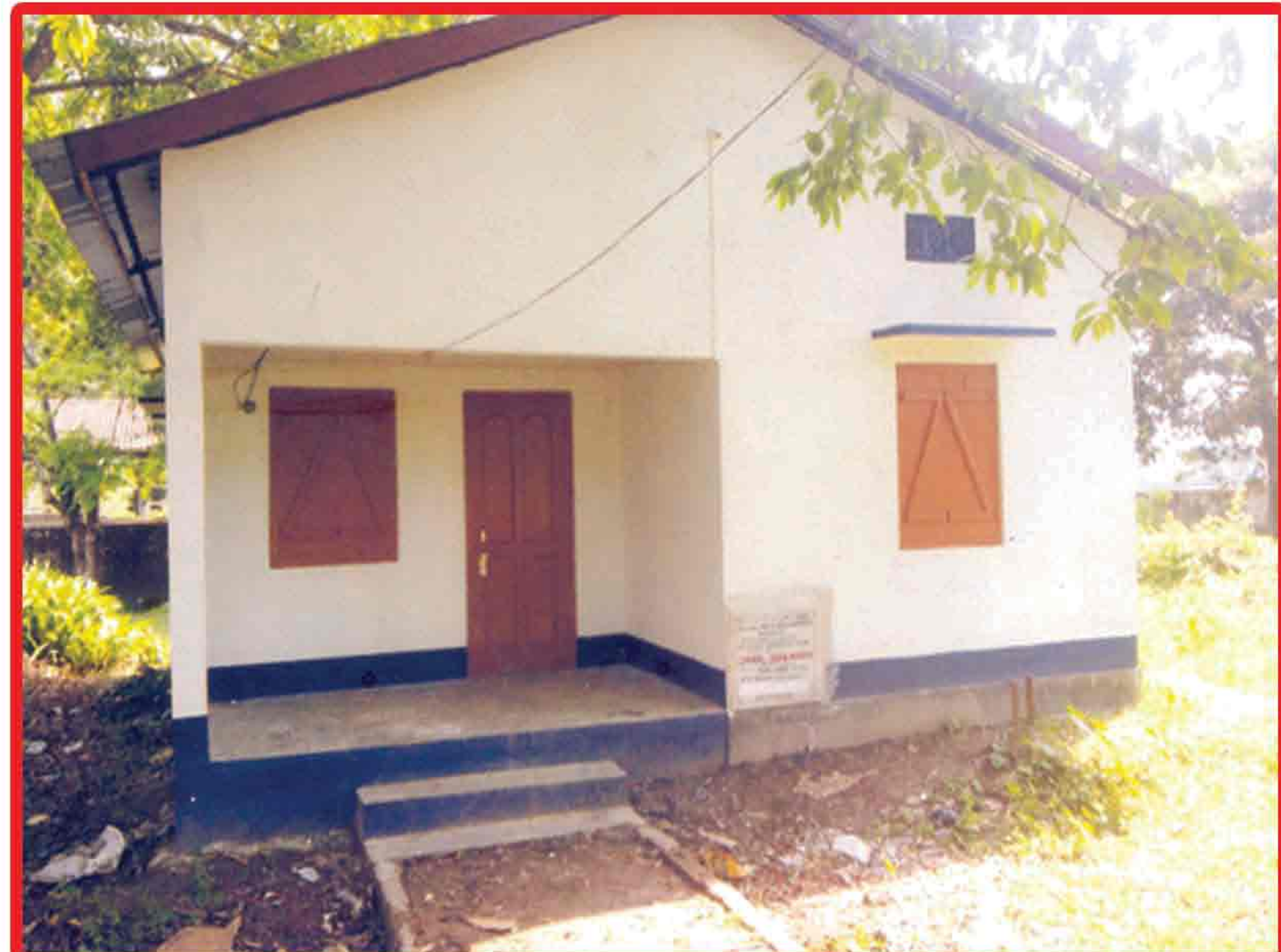
Construction of BDO/E.O Quarter at Badarpur A.P.
