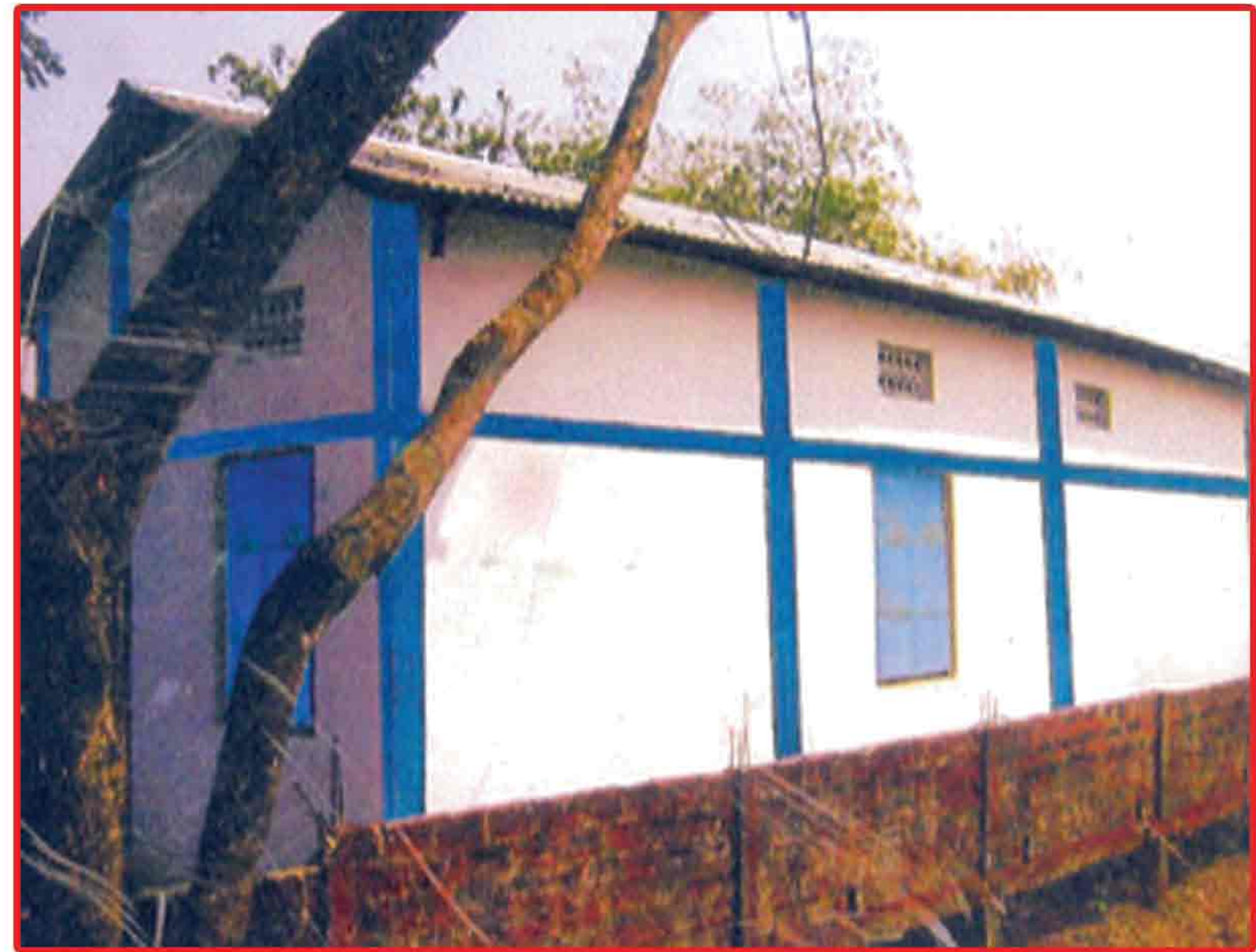
Construction of G.P. Secy Quater at Hasanpur G.P.
