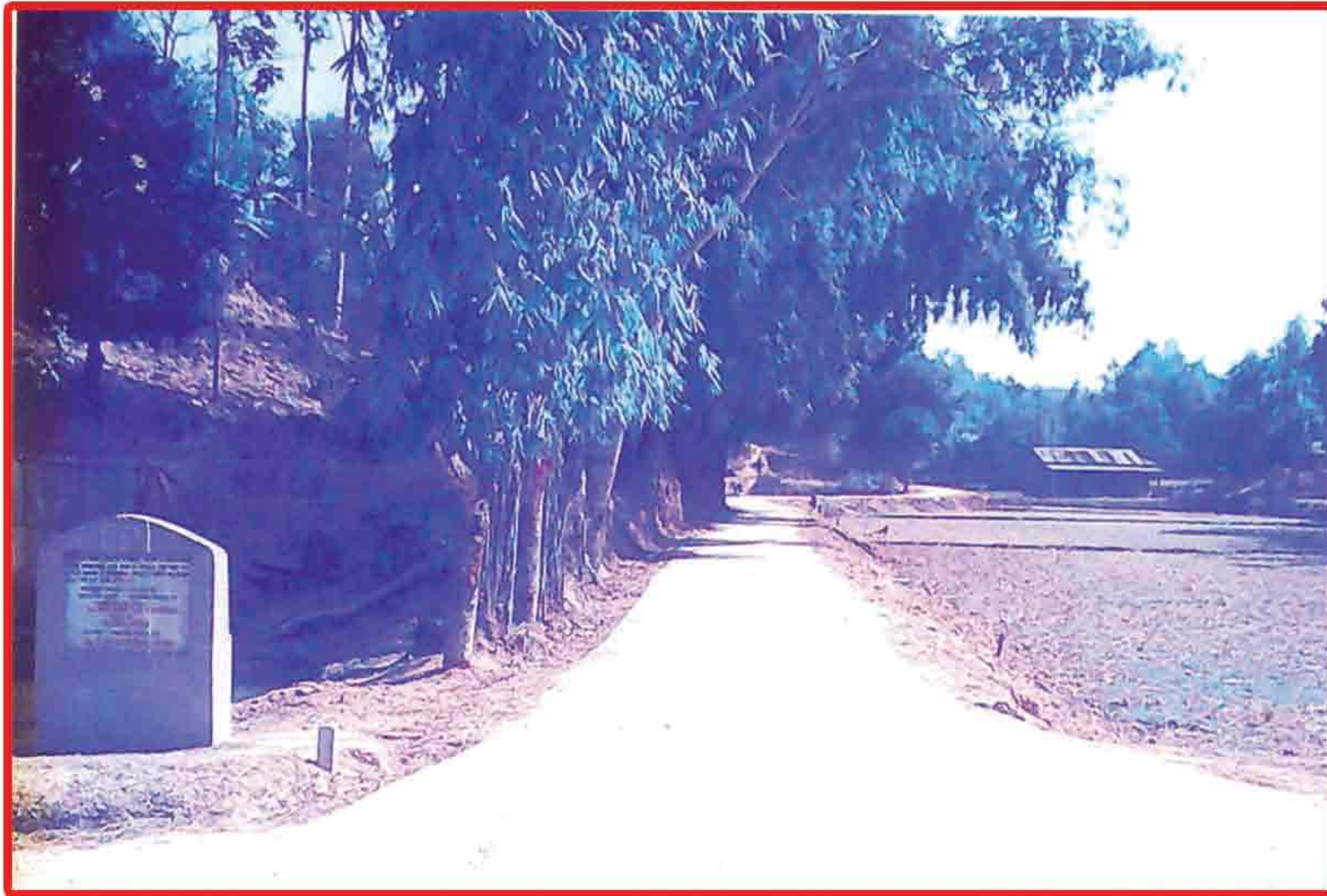
Const. of Road with Brick Salling From Manikpara P.W.D. Road to Duhalia MNP via Utlan Maszid at Vill- Manikpar.
