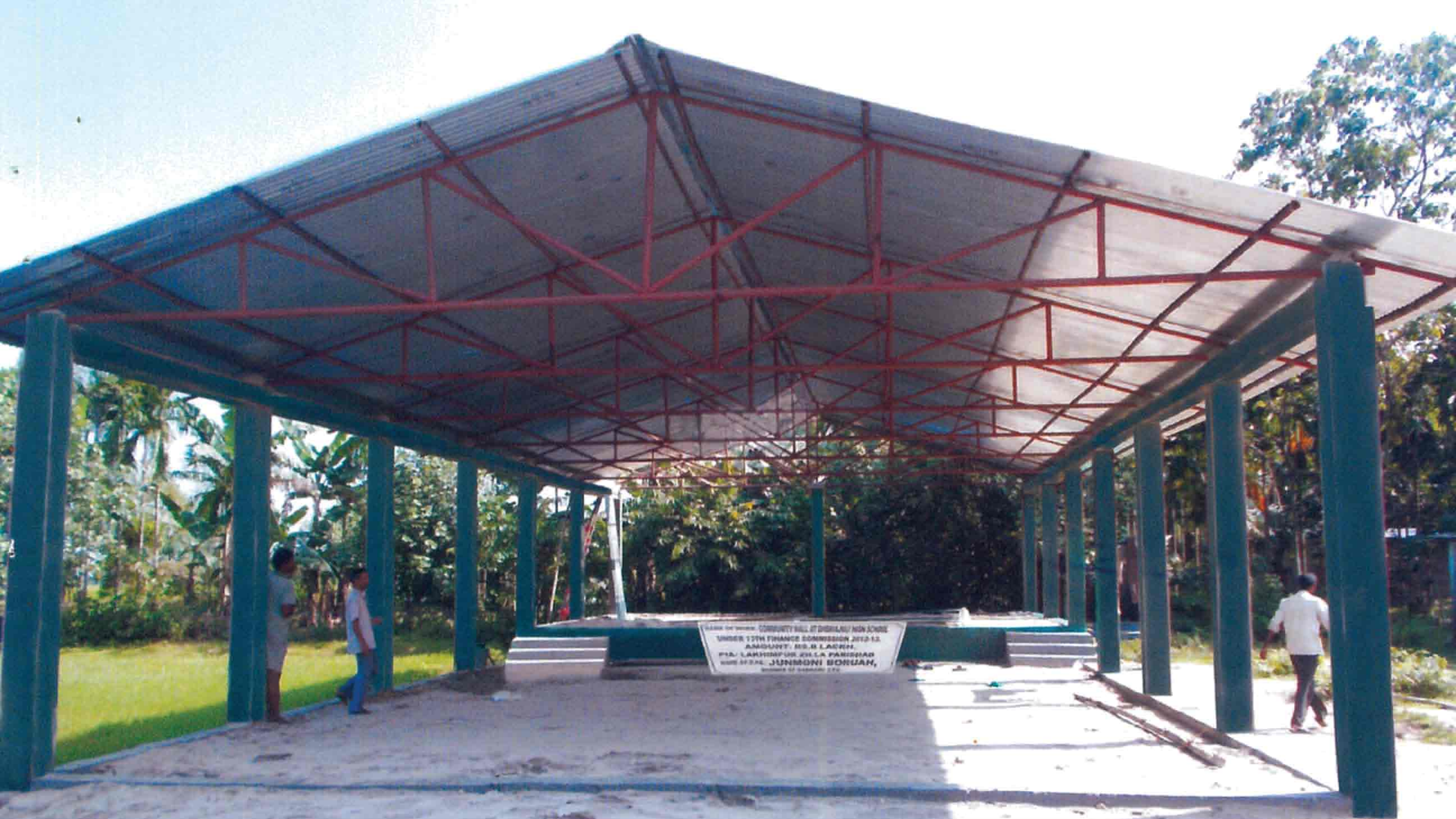
CONSTRUCTION OF COMMUNITY HALL AT DHEKIAJULI H.S.,UTTAR LALUK G.P. UNDER 13 TH F.C. FOR THE YEAR 2012-13 Estimated Amount - 8.00(L) PIA Lakhimpur Zila Parishad
