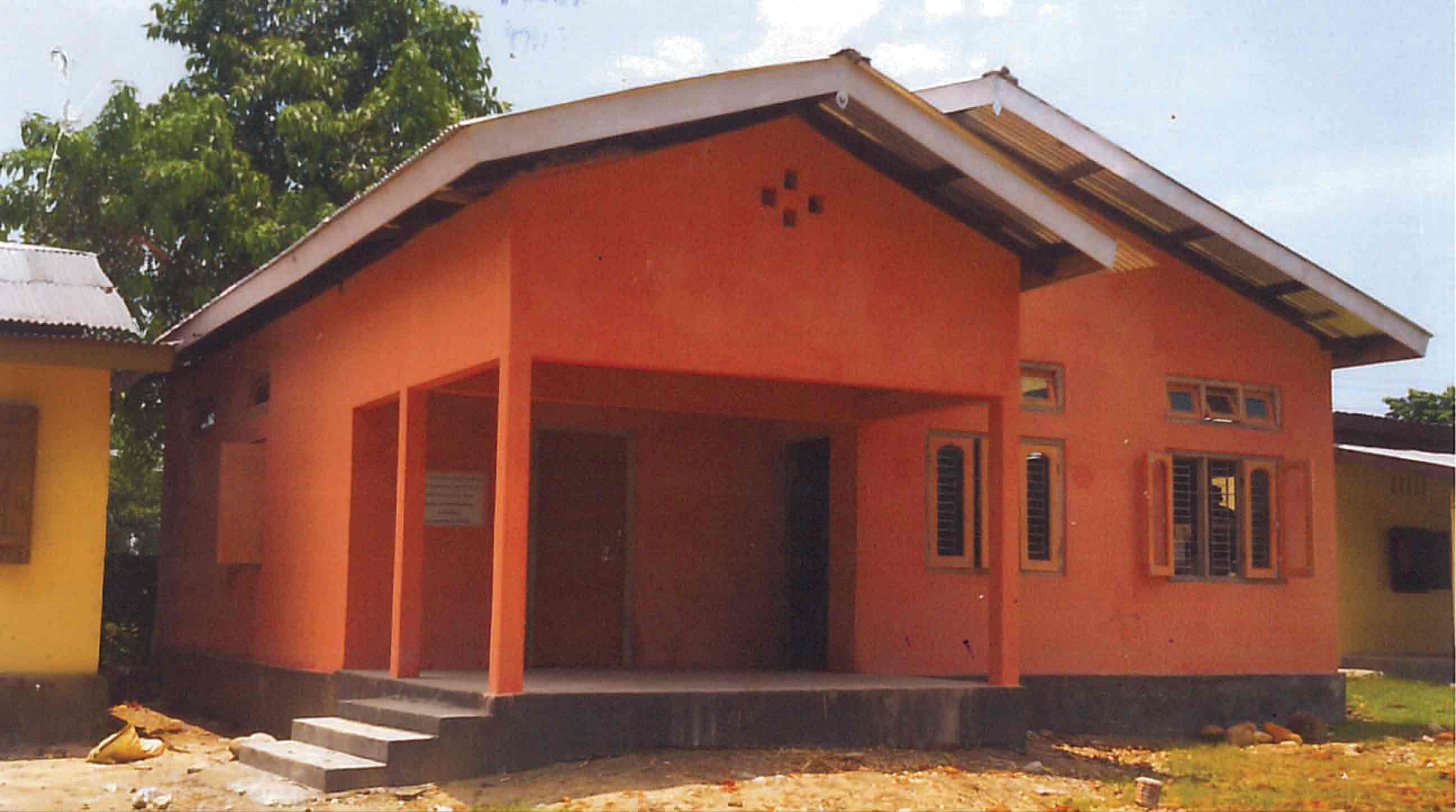
CONSTRUCTION OF COMMUNITY HALL NEAR BOGINADI POLICE STATION UNDER 13 TH F.C. FOR THE YEAR 2012-13 Estimated Amount - 8.00(L) PIA Lakhimpur Zila Parishad
