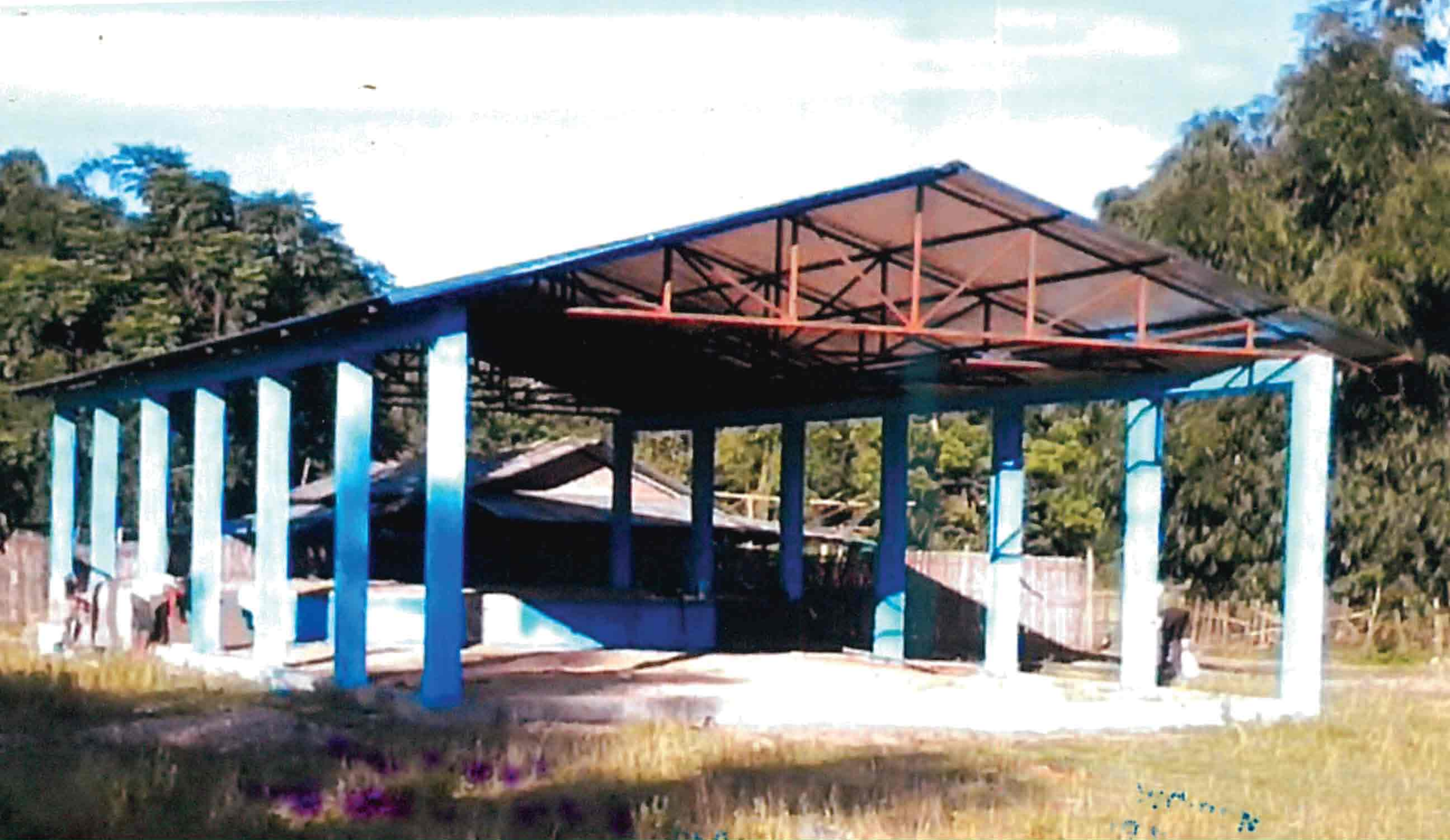
CONSTRUCTION OF COMMUNITY HALL SEYAJULI G.P. OFFICE CAMPUS UNDER 13 TH F.C. FOR THE YEAR 2012-13 Estimated Amount - 8.00(L) PIA Lakhimpur Zila Parishad
