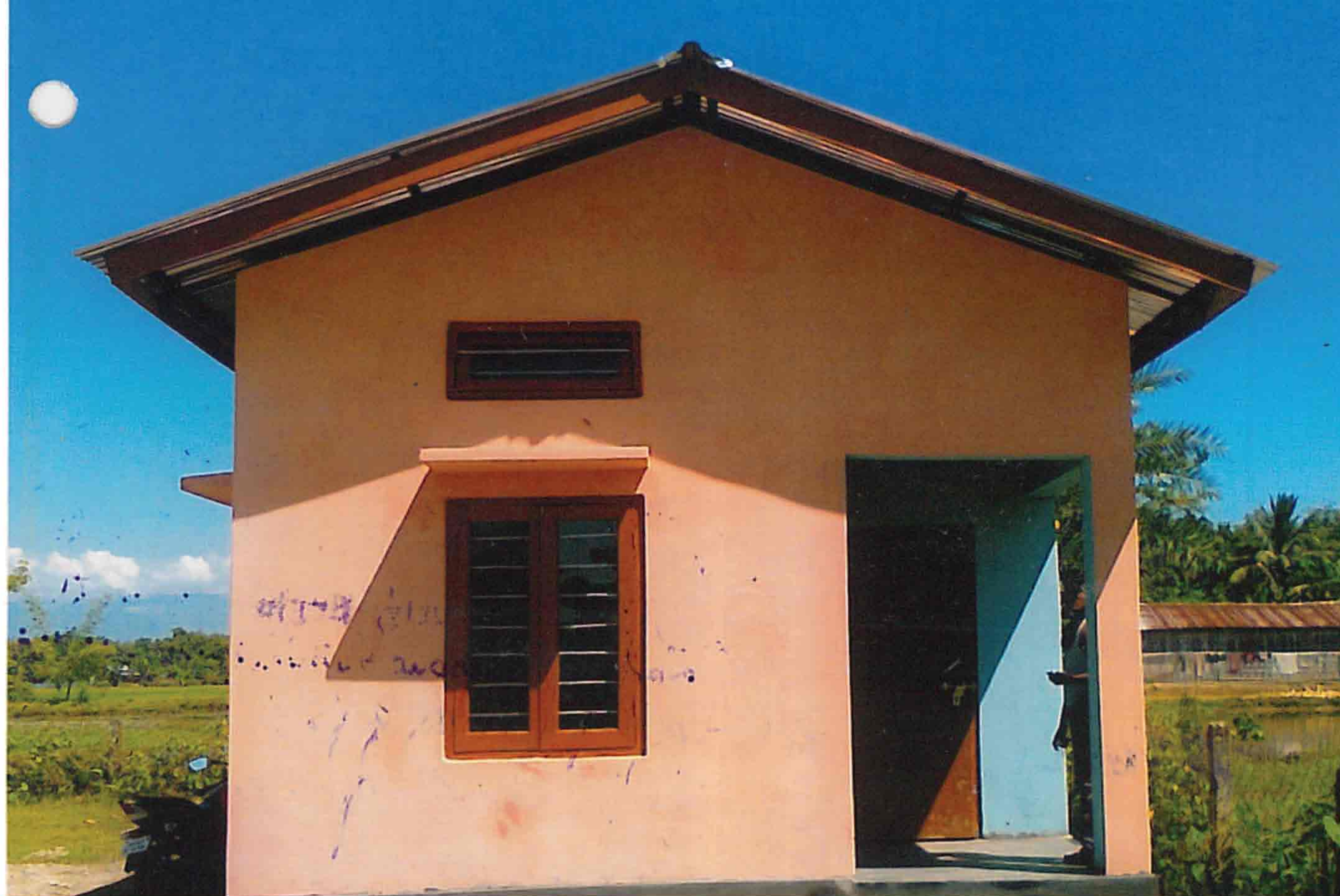
CONSTRUCTION OF G.P. SECETARY QUARTER AT PAVA G.P. OFFICE CAMPUS UNDER FASFC FOR THE YEAR 2011-12 Estimated Amount -3.40(L) PIA Lakhimpur Zila Parishad
