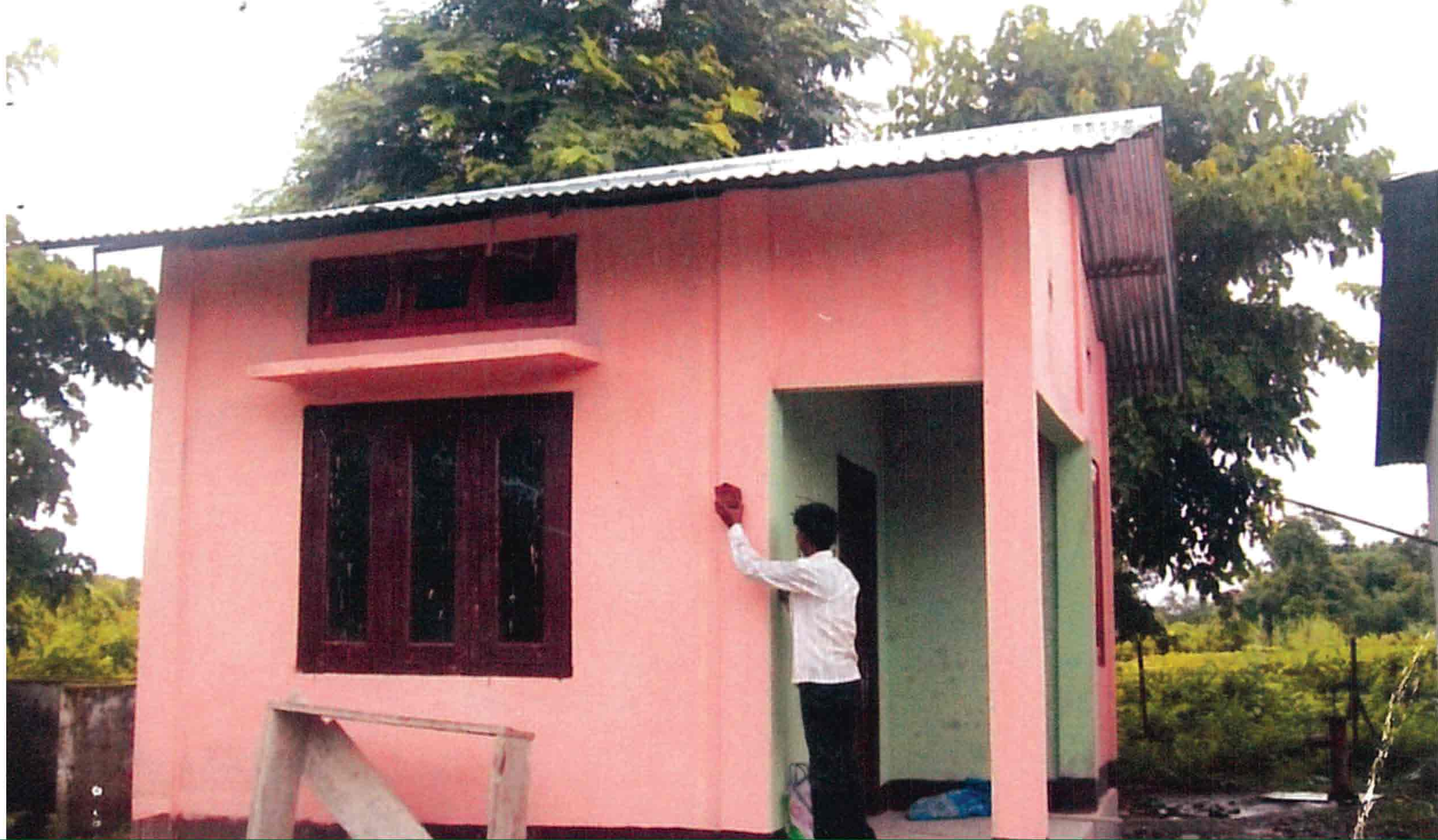
CONSTRUCTION OF GRADE -IV QUARTER AT UTTAR DHAKUWAKHANA G.P. OFFICE CAMPUS UNDER FASFC FOR THE YEAR 2011-12 Estimated Amount - 2.10(L) PIA Lakhimpur Zila Parishad
