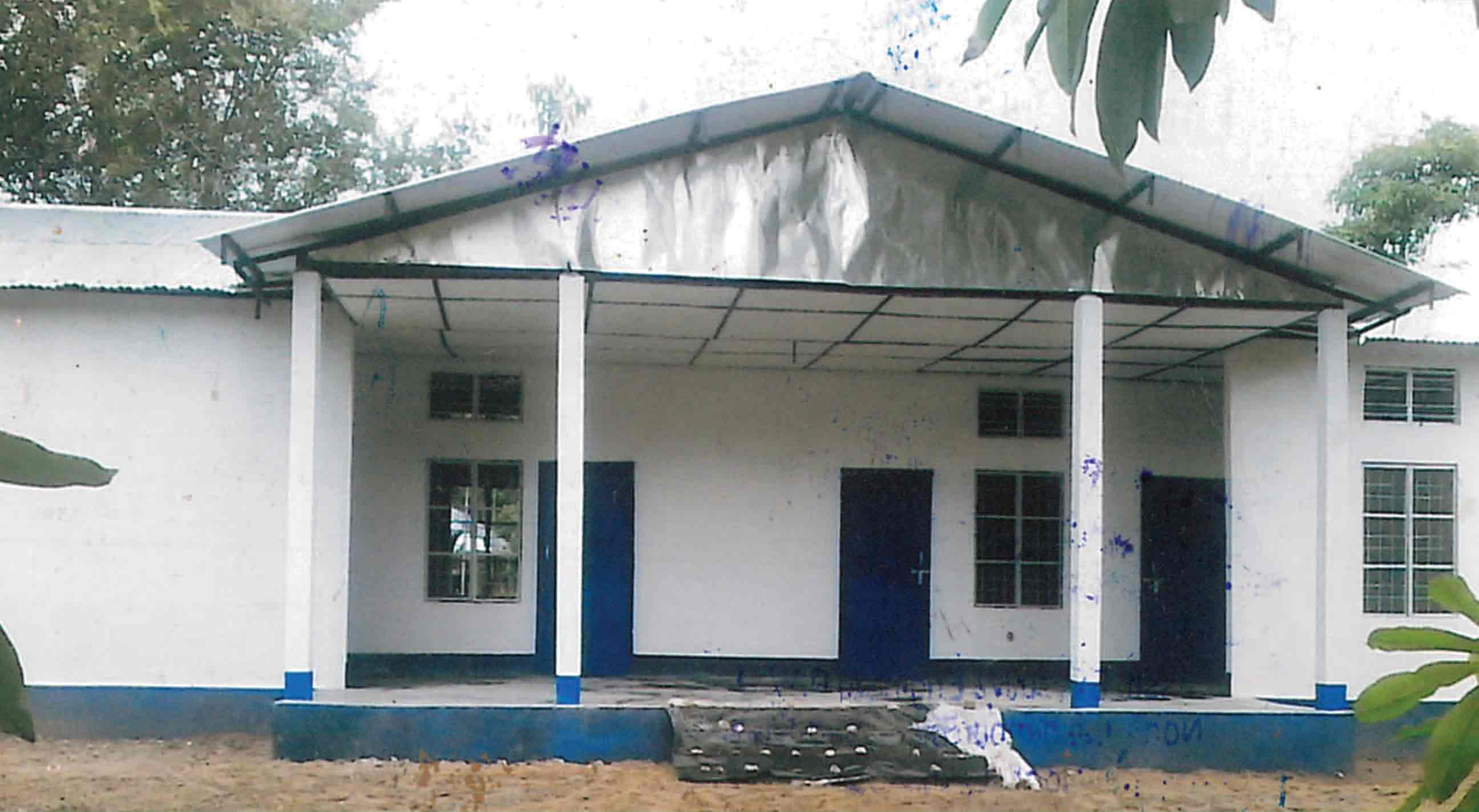
CONSTRUCTION OF G.P. OFFICE BUILDING AT UJJALPUR G.P. OFFICE CAMPUS UNDER FASFC FOR THE YEAR 2011-12 Estimated Amount - 11.00(L) PIA Lakhimpur Zila Parishad
