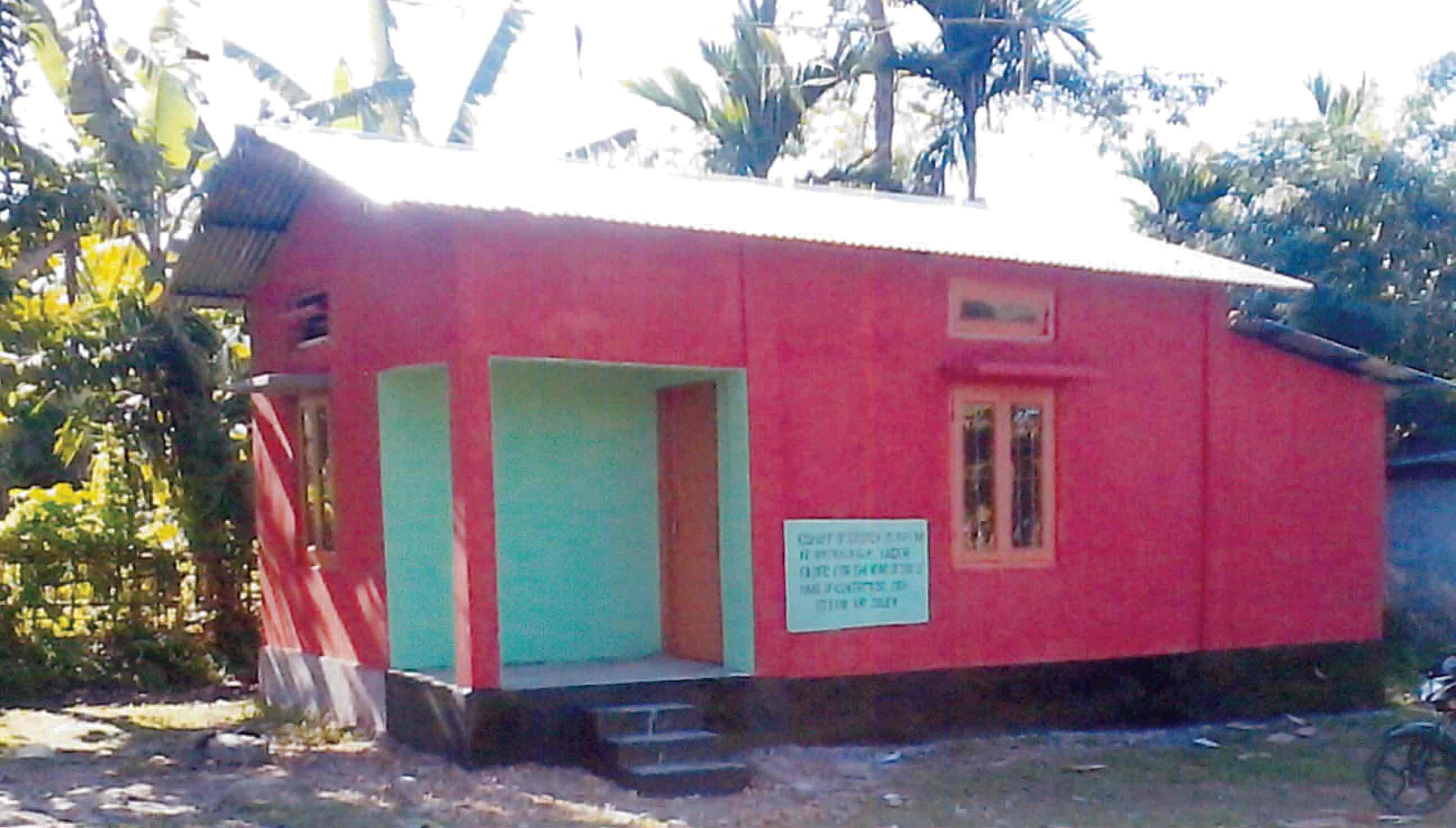
CONSTRUCTION OF G.P. SECETARY QUARTER AT MATMORA G.P. OFFICE CAMPUS UNDER FASFC FOR THE YEAR 2011-12 Estimated Amount -3.40(L) PIA Lakhimpur Zila Parishad
