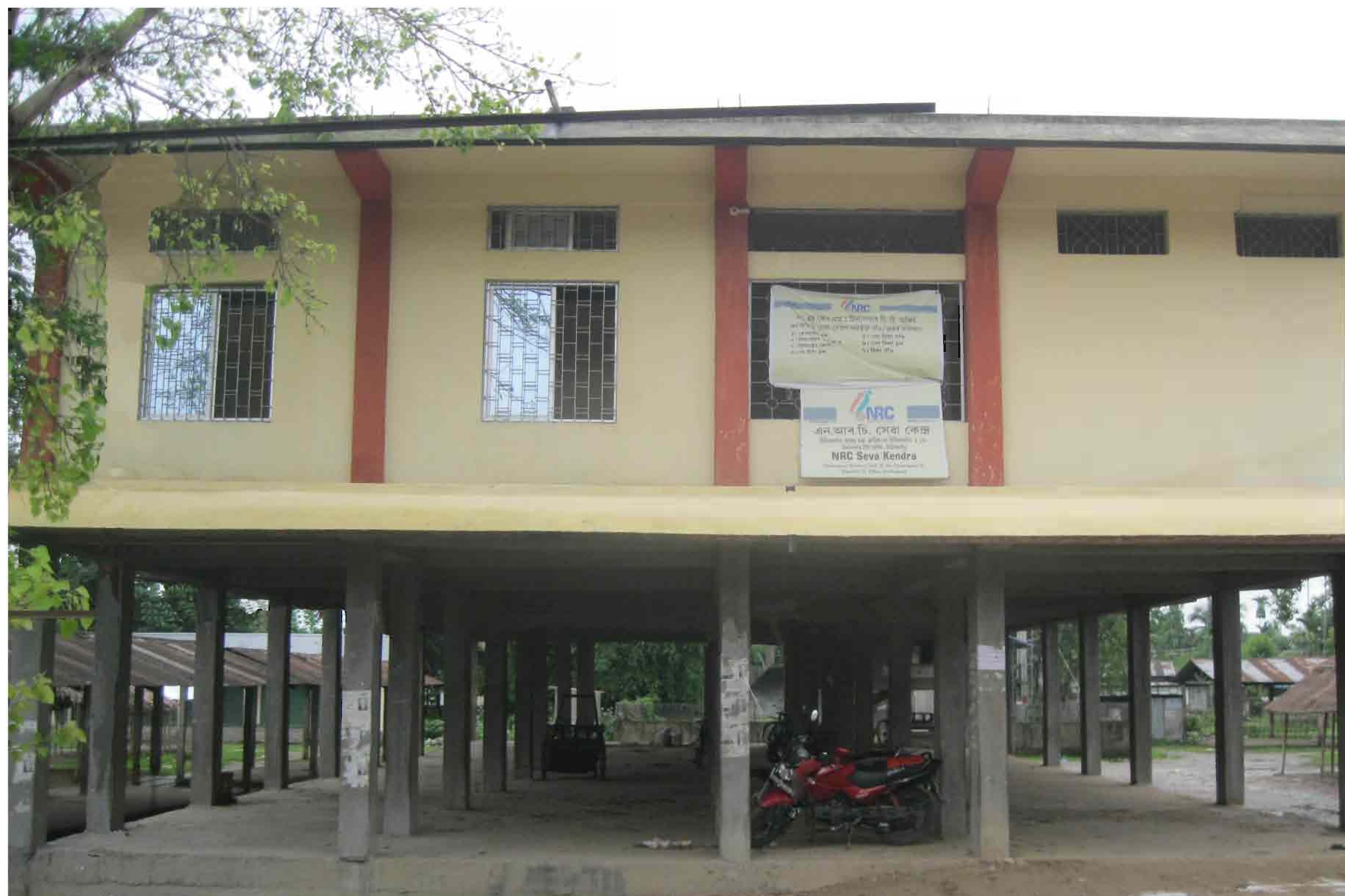
Name of Scheme:- Construction of Office Building of Silapathar Town Committee & Market Complex under 4 th Assam State Finance Commission- 2011-12.
