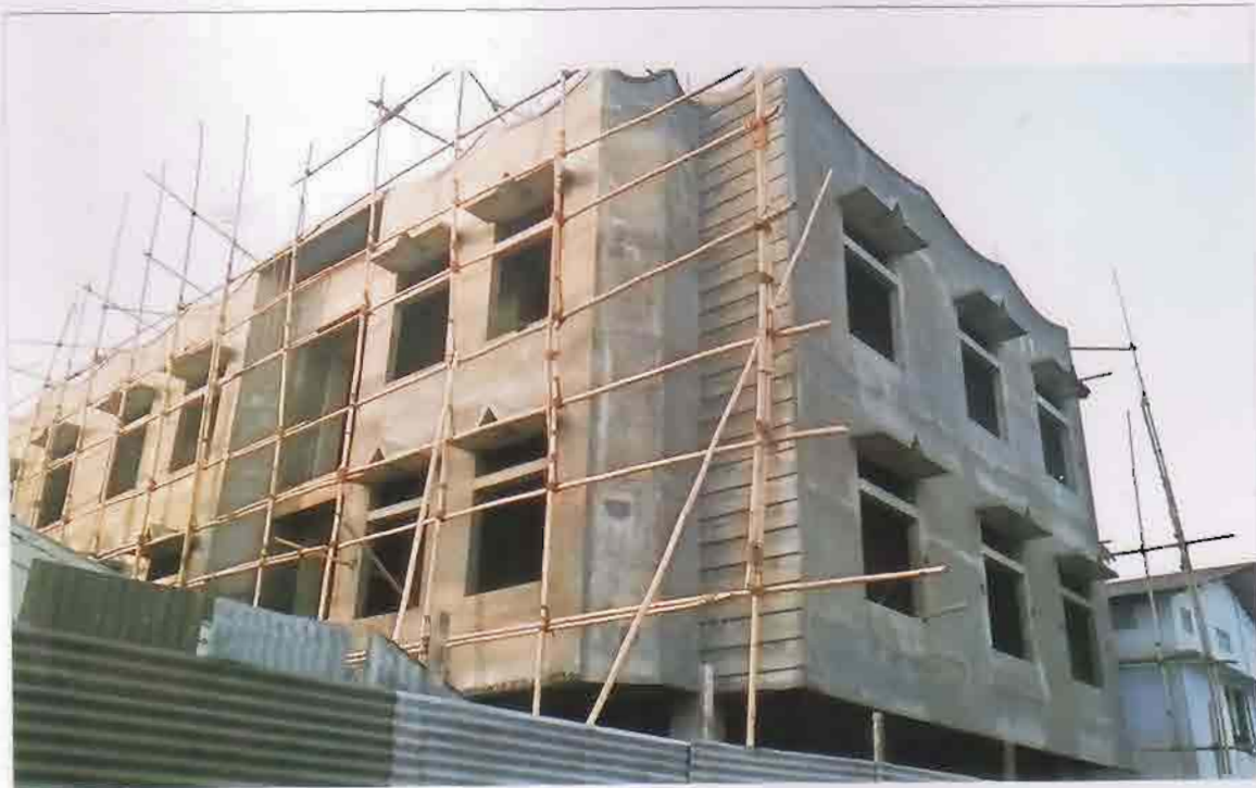
PLASTERING WORKS IN OUTER WALL OF BUILDING (WORK IN PROGRESS)
