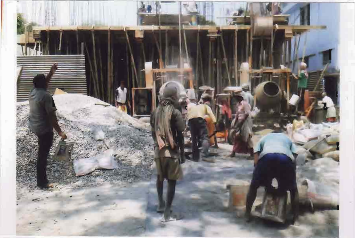
SLAB CASTING OF GROUND FLOOR (WORK IN PROGRESS)
