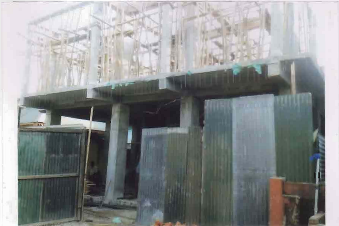
FORM WORK FOR SLAB CASTING OF 1ST FLOOR (WORK IN PROGRESS)
