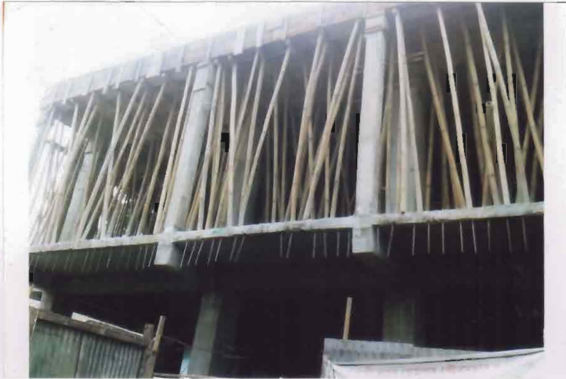
AFTER SLAB CASTING OF 1ST FLOOR (WORK IN PROGRESS)
