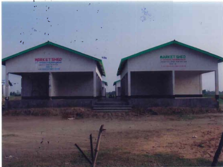
Market shed at Hatishola Deoboria Bazar in Goroimari ZPC under XIII Finance Commission 2012-13(1st instt.)
